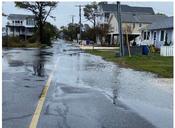
Figure 2.1. Inundation of York Road just south of the intersection with Plymouth Road during a typical rainfall.
