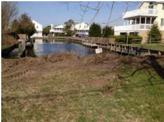
JUNNIPERS AND ROOTS REMOVED
